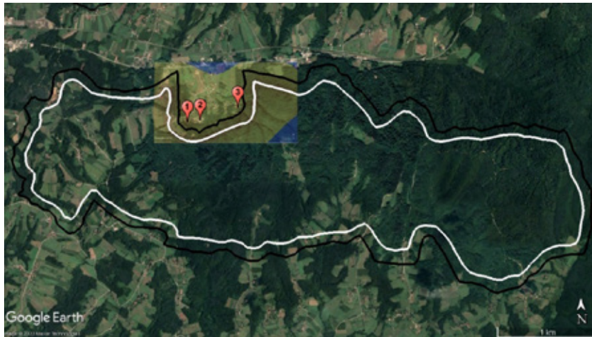
Figure 2. The first examined segment of the mine front, 2317 m long, with proposed measuring points, next to residential areas near the potentially most affected by emitted noise from heavy machinery
